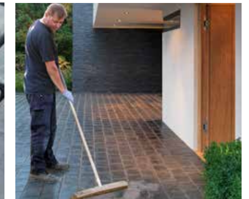
6. Brush in Stonemarket Driveway Jointing Compound following the instructions on the tub, using plenty of water
