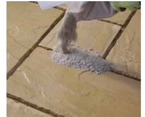
3. The Fast Point jointing is poured onto the paving after soaking
