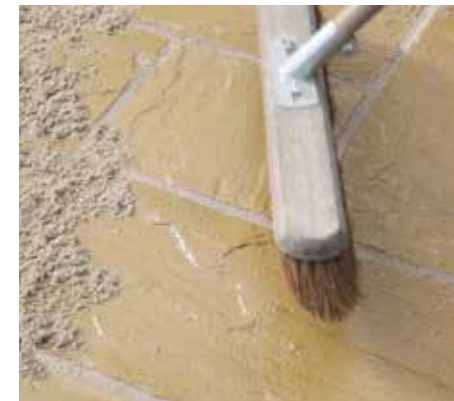
4. The material is brushed into the joints ensuring the joint voids are full
