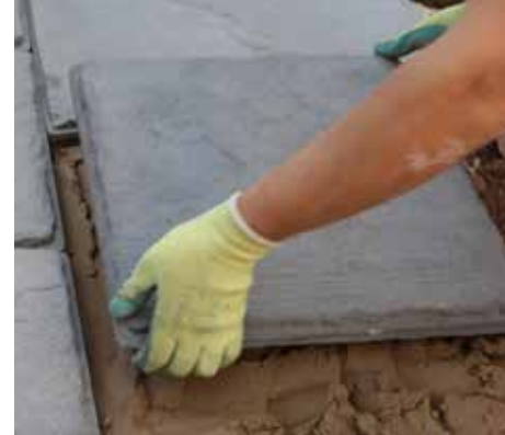
4. Install the engineered NEXTpave using the laying pattern
