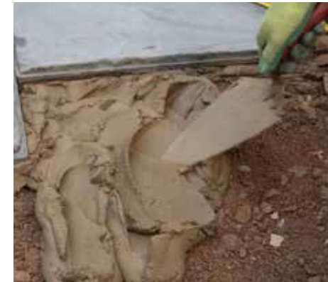
3. Install the engineered NEXTpave flags onto a full bed of mortar; 1 part cement to 5 parts building sand.
