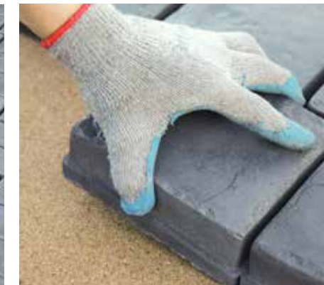
5. Make a solid connection when laying the blocks to ensure a perfect uniform joint
