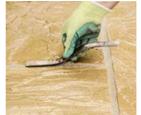
6. The joints are struck off using a pointing iron. Any gaps that are revealed, re fill with Fast Point
