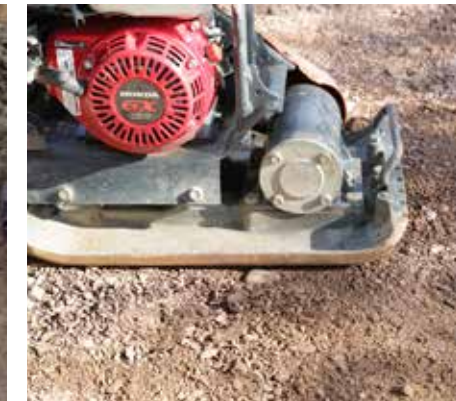
2. Prepare the ground as normal with compacted hardcore, achieving the correct falls for drainage
