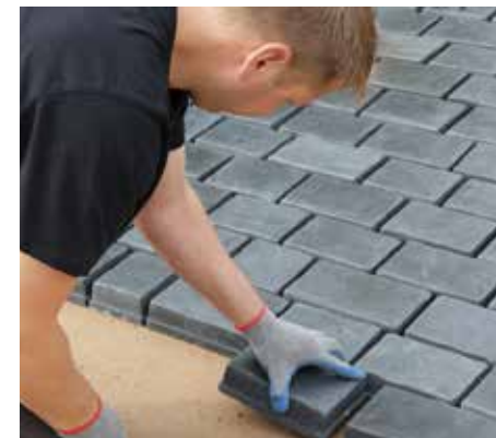
4. Install the engineered Templeton or Millstone Driveway Setts
