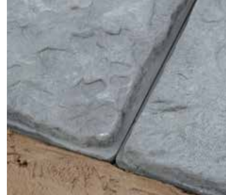
5. Make a solid connection when laying the NEXTpave to ensure a perfect uniform joint
