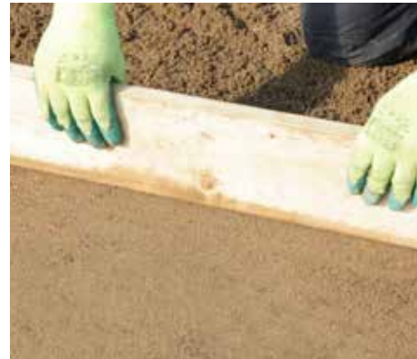
3. Screed out a 30-40mm sharp sand bed
