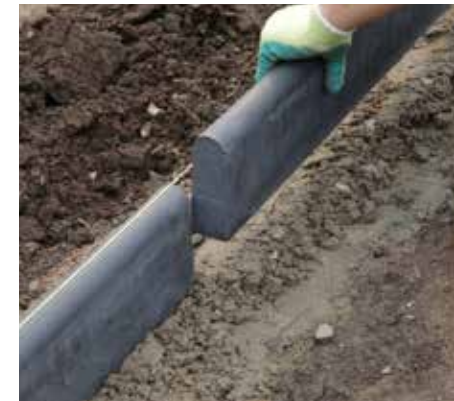
1. Install your choice of edge restraint on a concrete footing around the perimeter of the driveway
