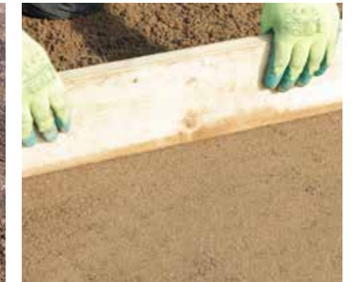
3. Screed out a 30mm sharp sand bed
