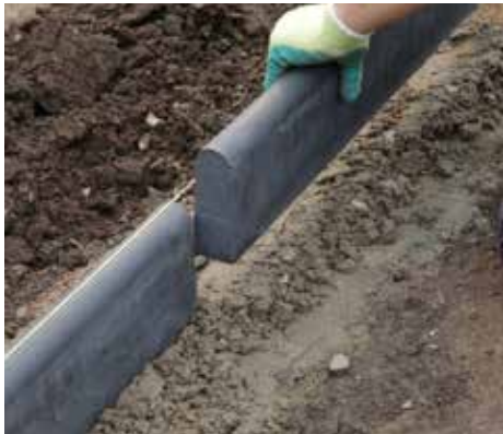
1. Install your choice of edge restraint on a concrete footing around the perimeter of the patio
