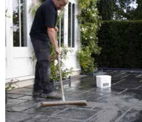
6. After 24 hours brush in Stonemarket FastPoint following the instructions on the tub, using plenty of water
