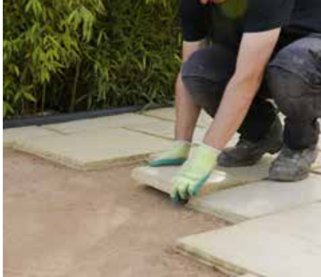
4. Install the engineered NEXTpave using the laying pattern
