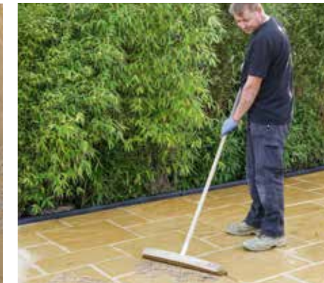
5. Any excess is carefully brushed off. Particles left on the paving may leave a speckled finish.
