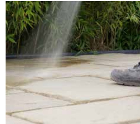
1. The paving is soaked with a hose. Keep wet throughout process to avoid any temporary staining
